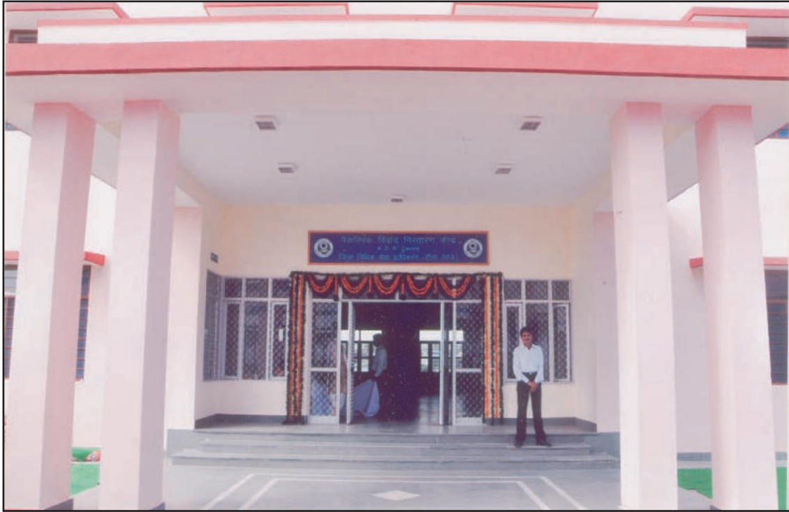
The newly constructed building of ADR Centre at Dausa.
